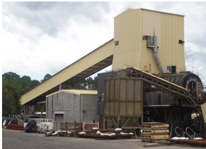
Plate 5 – Rotary Breaker at CCF
