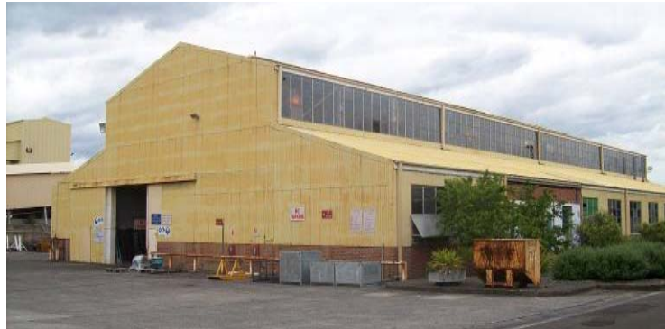
Plate 2 – Manning Colliery Workshop
