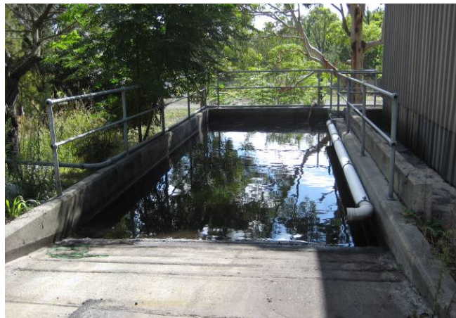
Plate 8 – Drive-In Sump at Manning Colliery
