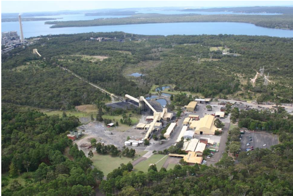
Plate 1 – Manning Colliery Surface Facilities
