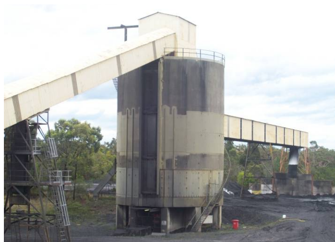
Plate 6 – Product Coal Stockpile Bin
